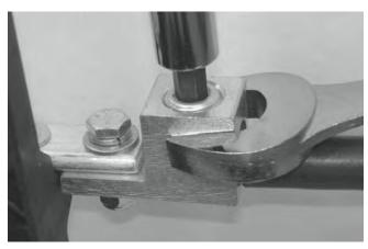
**Note:** When securing the lugs onto the bus bars of the soft starters, use a suitable tool such as another wrench to counteract the bolt torque and prevent excessive side loads being placed on the supports. Refer to figure "Lug and Bolt Torque Support" above.
